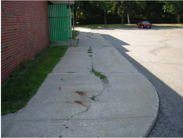
Damaged Concrete Walk
