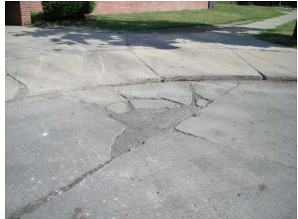
Damaged Asphalt Drive
