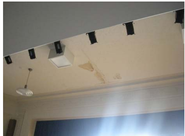
Water Damage at Auditorium Ceiling
