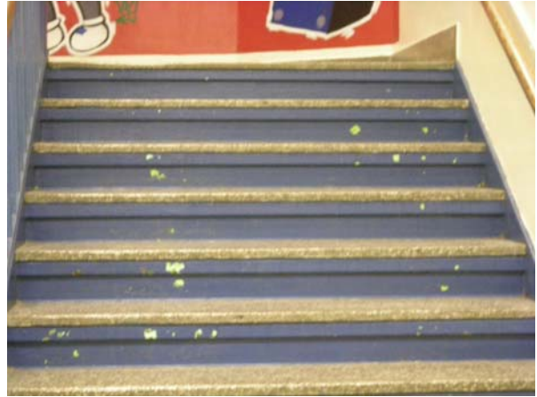
Chipped Paint at Metal Stair Risers
