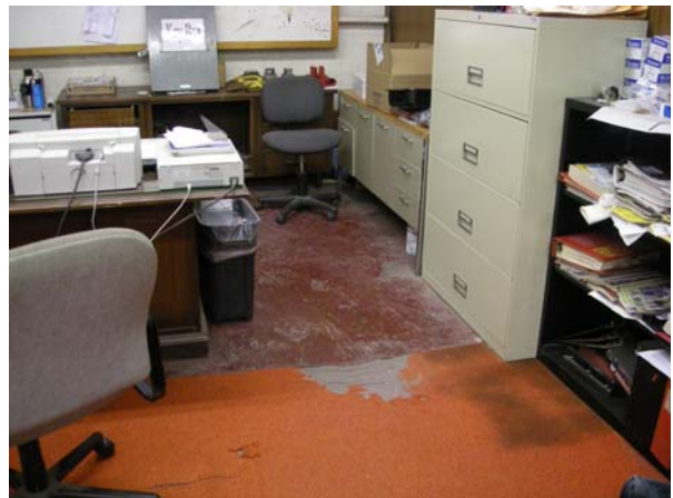
Worn and Missing Carpet
