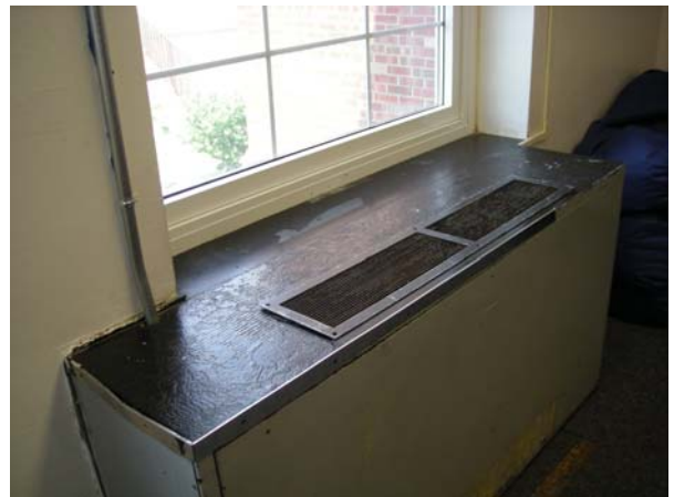
Typical Unit Ventilator
