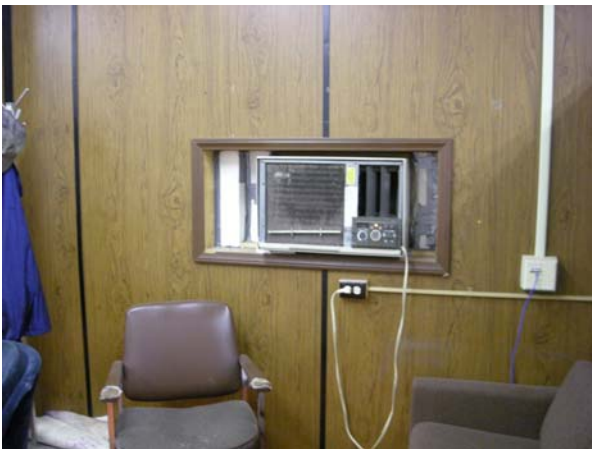
Custodian's AC draws air from Boiler Room
