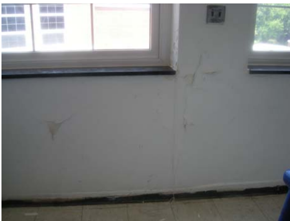
Plaster Damage
