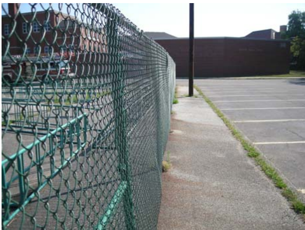
Damaged Chain Link Mesh
