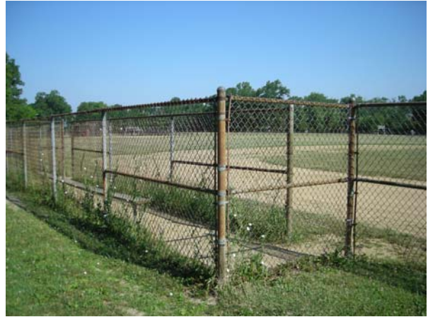
Deteriorated Chain Link Fence
