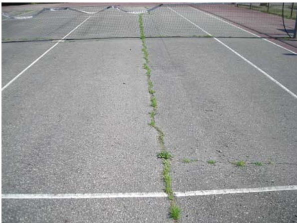
Tennis Court Damage
