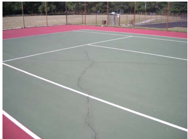
Tennis Court Damage
