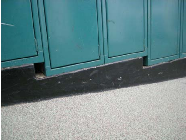
Gaps at Locker Base
