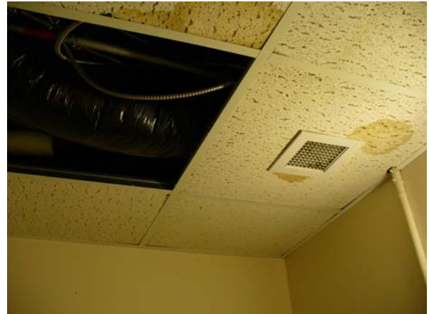
Lay-In Ceiling Damage
