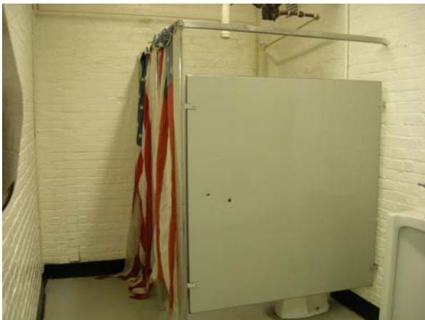
Missing Toilet Partition Doors
