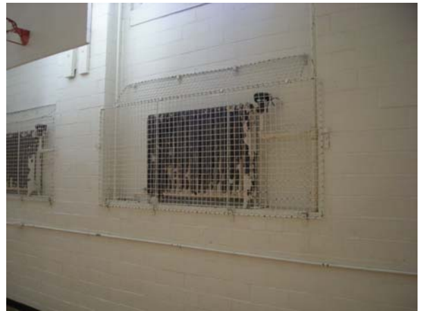
Obsolete Radiator in Gymnasium
